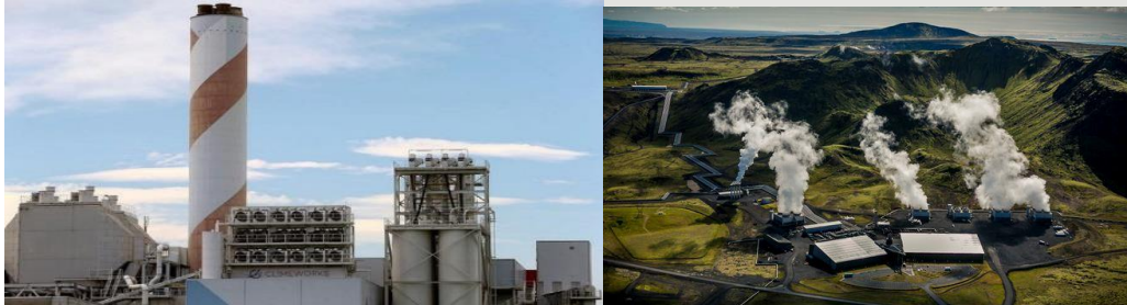
Figure VI: Climeworks DAC Facility, Switzerland and Iceland.
